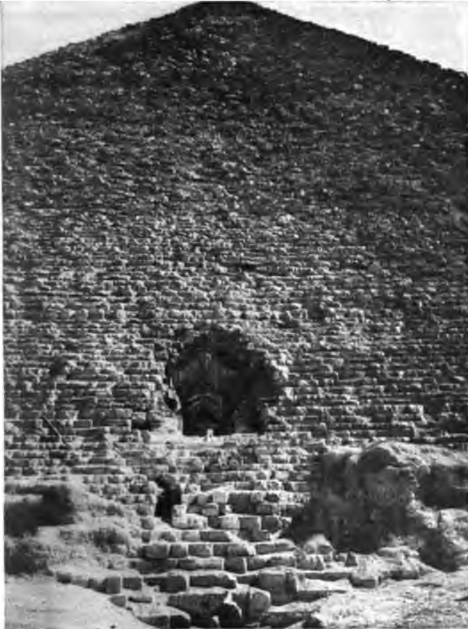
NORTH FACE OF THE GREAT PYRAMID, SHOWING THE ENTRANCE.
